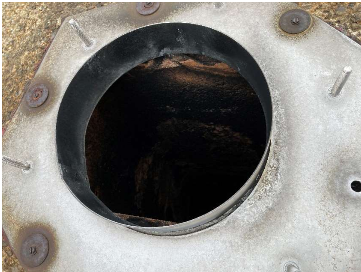
Picture 11: Missing chimney hood above base cap.
