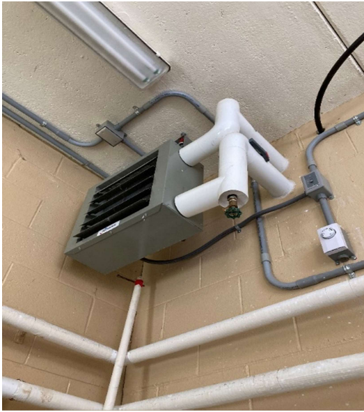
Pictures 8 and 9: Modine suspended unit heaters in the Headworks Building.
