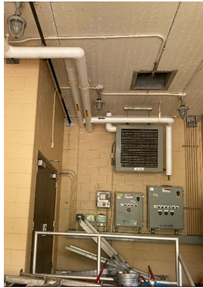
Pictures 8 and 9: Modine suspended unit heaters in the Headworks Building.
