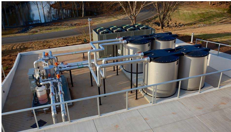
Picture 14: A Trane TES insulated outside tank system for a larger facility.
