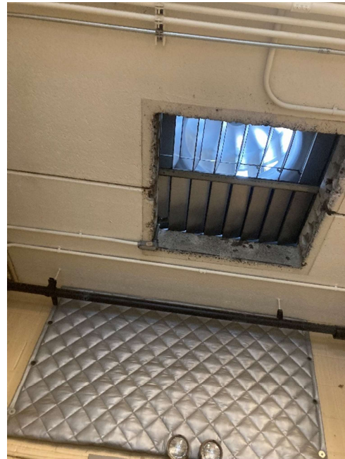
Picture 18: Roof air inlet shutter for Blower Room.
