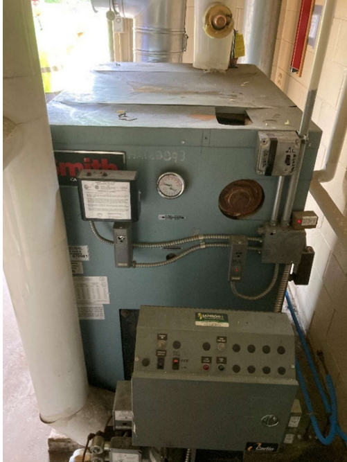
Pictures 4 and 5: The front and rear views of the Headworks Building's Smith hydronic boiler.
