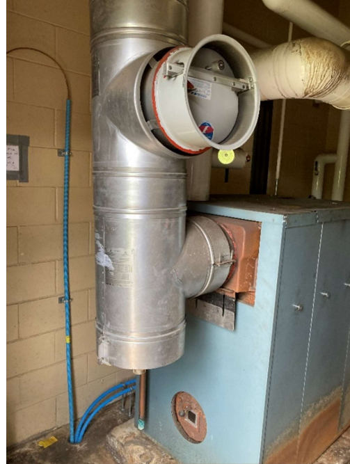
Pictures 4 and 5: The front and rear views of the Headworks Building's Smith hydronic boiler.
