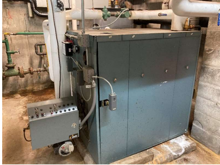
Picture 10: The oil-fired, Smith cast iron boiler in the Process Building basement.
